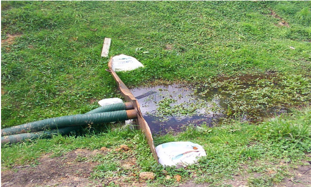
Photo 8.2 Metal plate weir used as a temporary dam to divert flows around the working area (Photo: Wood & Partners Ltd)
