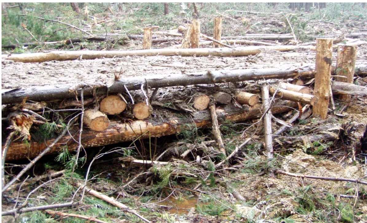
Photo 8.1 Example of a temporary log crossing over an ephemeral gully with a small upper catchment
